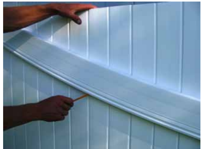
4. Trace the Outline of the Rail onto the Pickets
