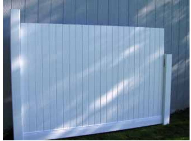
2. Insert Pickets in Bottom Rail
